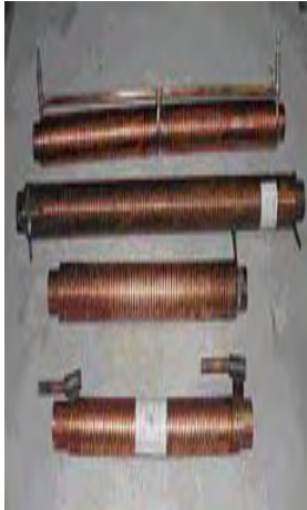
Figure 1 – Typical drain water heat recovery devices
