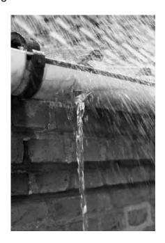
**Downspouts**. The rule of thumb for downspouts: at least one downspout for each 40 feet (12 m) of gutter. For roofs with gutters, make sure that downspouts discharge so water will drain away from the foundation. Downspouts can be checked for size. Seven square inches is generally the minimum except for
