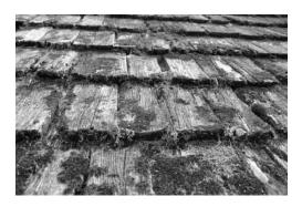
Wood shingles or shakes. This type of covering has a normal life expectancy of 20 to 30 years in climates that are not excessively hot and humid. Durability varies according to wood species, thickness, the slope of the roof, and whether shingles are made of heartwood. Maintenance may include periodically treating the covering with preservative.
