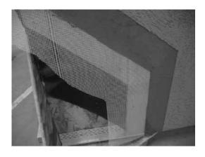
Stucco. Check stucco for cracks, crumbling sections and areas for potential water intrusion. Old and weathered cracks may be caused by the material's initial shrinkage or by earlier building settlement. New, sharp cracks may indicate movement behind the walls that should be investigated by a qualified professional. Stucco can be cleaned. It can also be painted.
