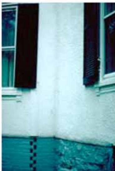
After thoroughly dampening the masonry or wood lath, the first scratch coat should be applied to the masonry substrate, or wood or metal lath, in a thickness that corresponds to the original (if extant), or generally about 1/4-inch to 3/8-inch. The scratch coat should be scratched or crosshatched with a comb to provide a key to hold the second coat. It usually takes 24 to 72 hours, and longer in cold weather, for each coat to dry
