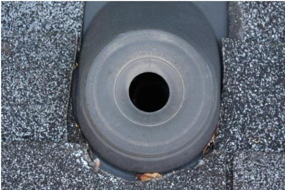
The vent pipe has been pulled downward approximately 1 ½ feet.
