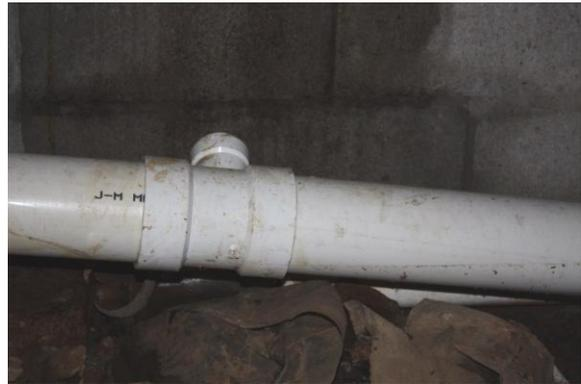
Vent stack coupling to the vent stack pipe. When the 6" PVC waste water line dropped, so did the vent stack pipe.
