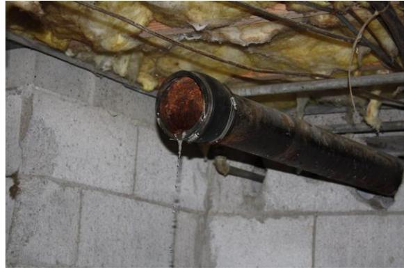
Cast iron pipe from utility/laundry area draining into the pool in the crawlspace.
