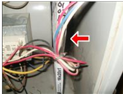
13.5 Picture 1 Damaged Filter
