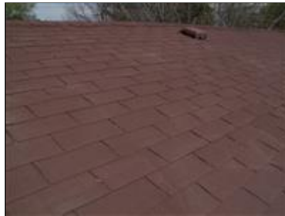
1.0 Picture 2 Painted Roofing
