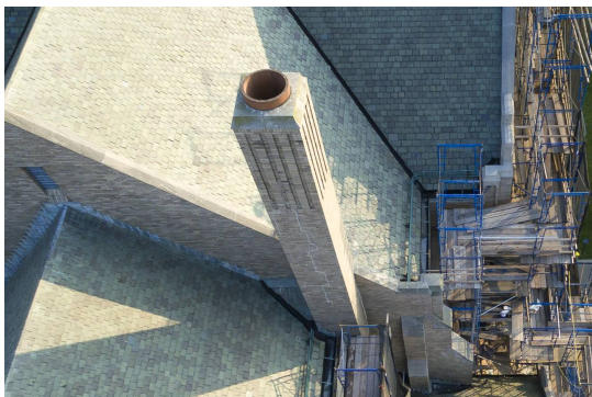
The chimney of a cathedral in Long Island, N.Y., could be inspected without having to erect scaffolds. PHOTO: ENGINEERED BUILDING INSPECTIONS
