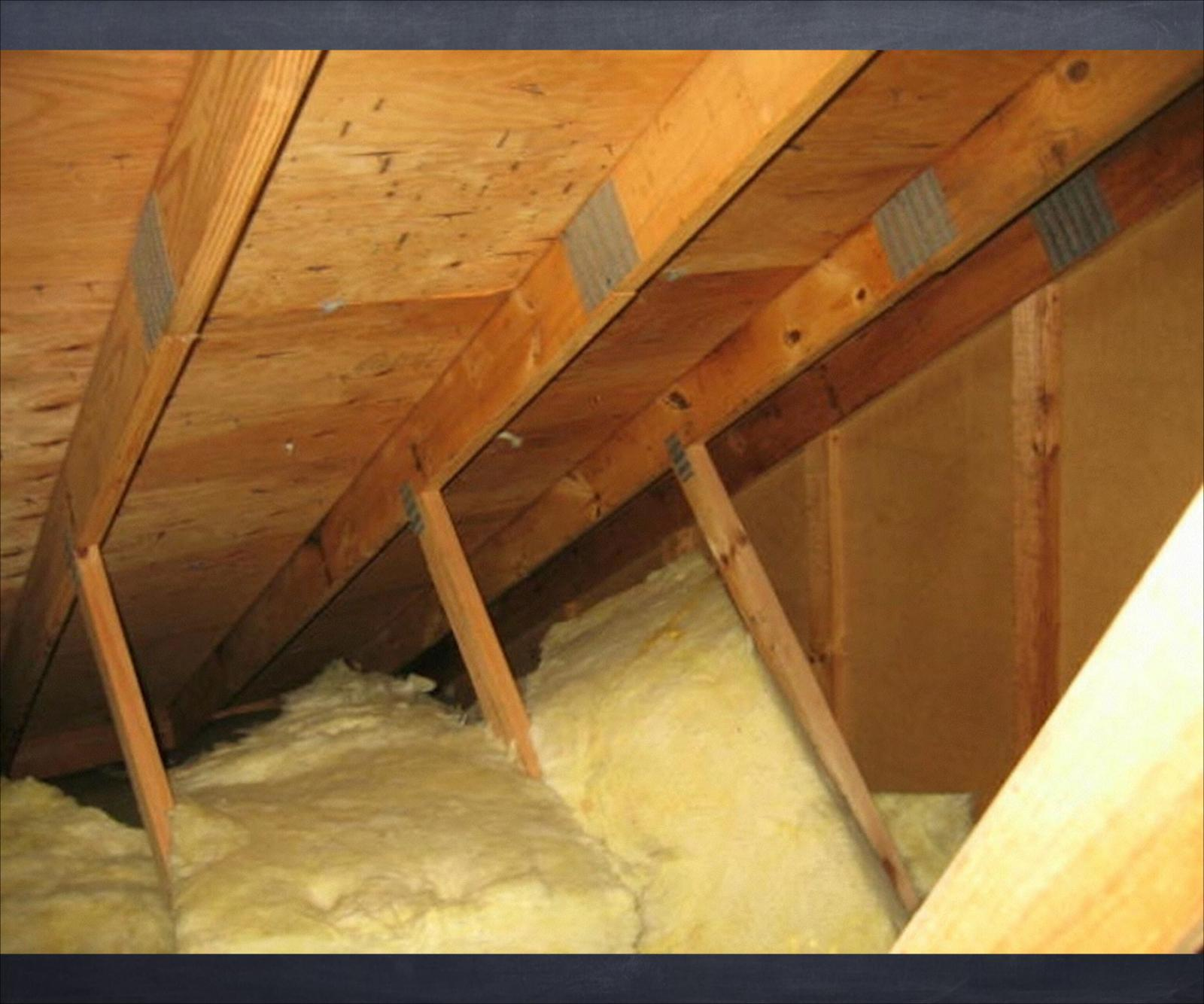
5. Panel spacer-type edge clips could be installed and recommended by some manufacturers.
