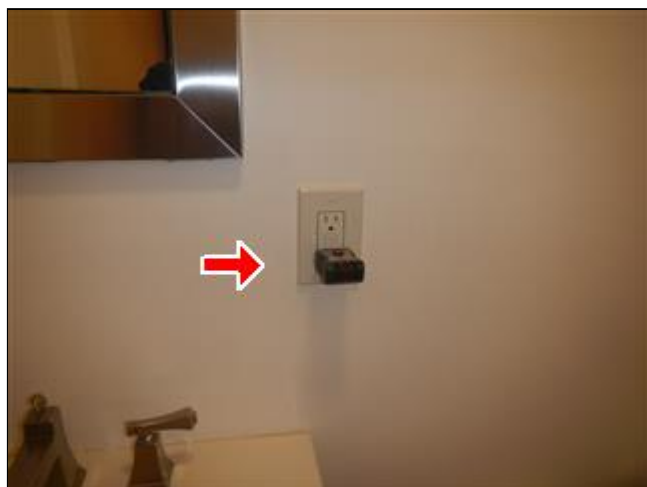
5.5.B Picture 1 Outlet has no current
