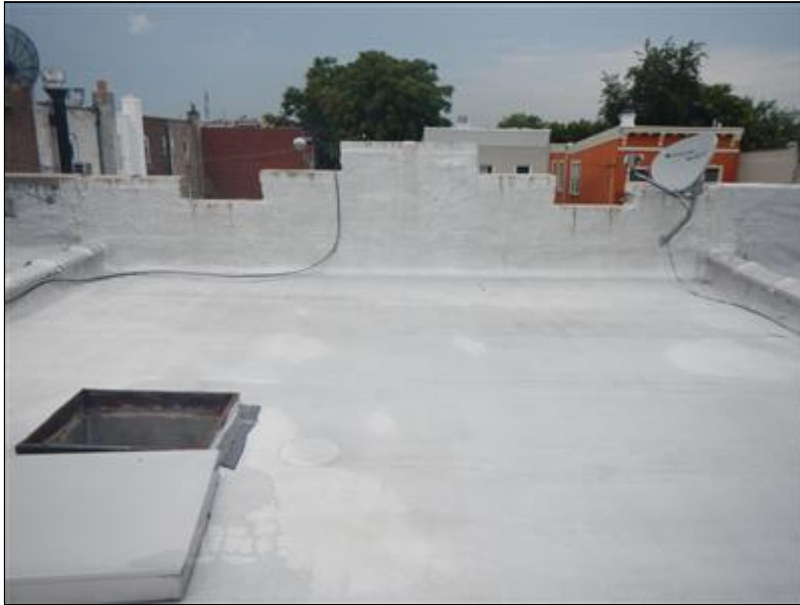
1.3 Picture 1 Roof View toward front, no vents visible
