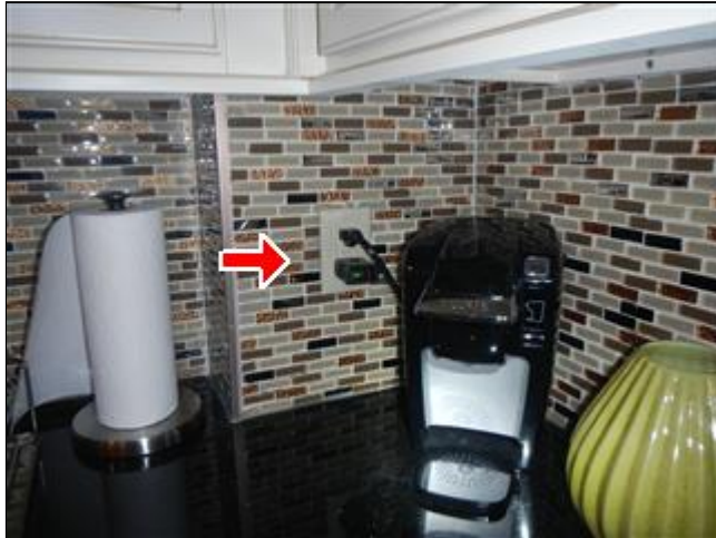
3.8.A Picture 1 Outlet to right of sink open ground
