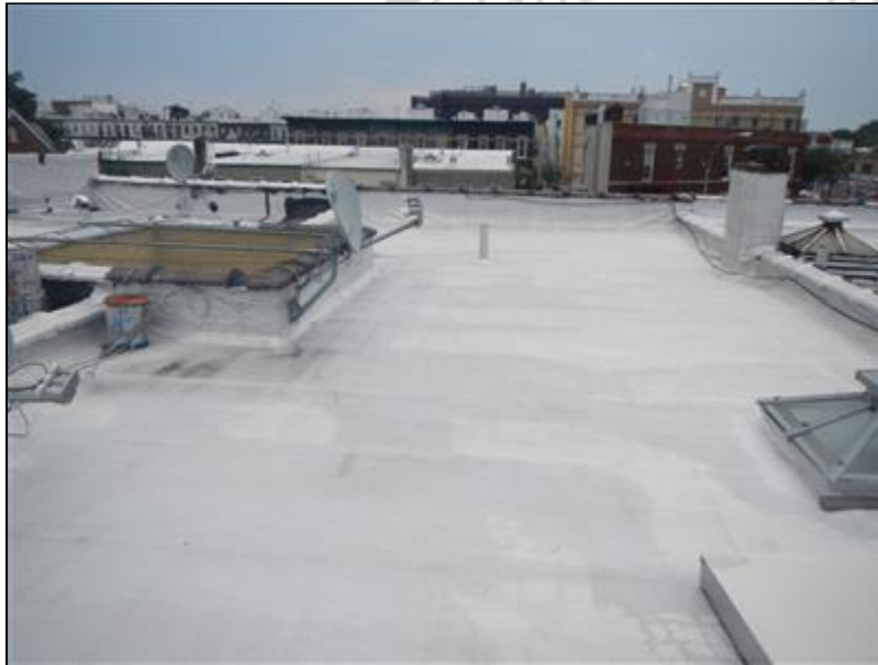
1.3 Picture 2 Roof View toward rear, no vents visible
