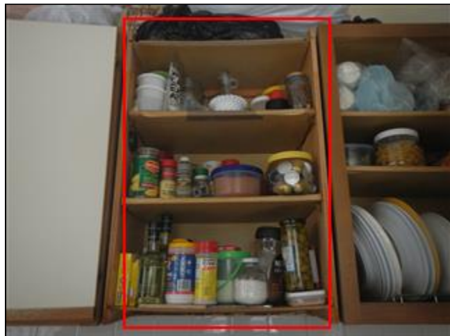
3.4.B Picture 1 Wall cabinet over sink style and door not attached
