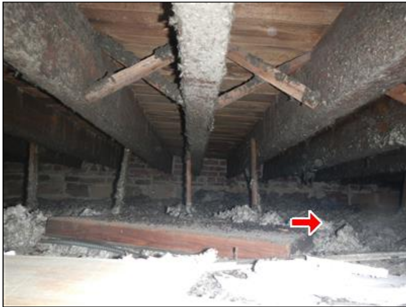
1.7 Picture 1 blown in insulation
