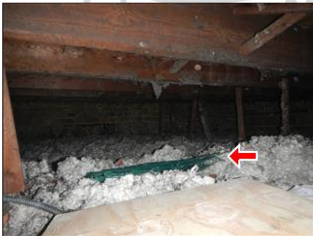
1.7 Picture 3 blown in insulation
