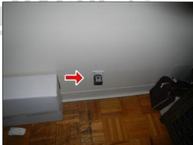
4.6.A Picture 1 Outlet open ground on right side
