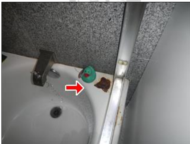
5.4.A Picture 1 Large rusted porcelain chip on bathtub flange
