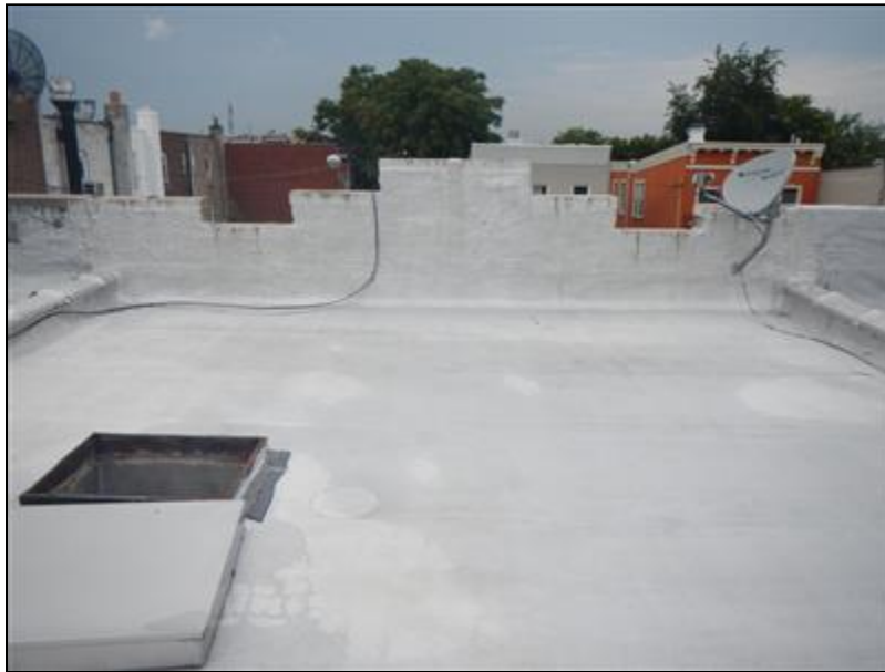
1.3 Picture 1 Roof View toward front, no vents visible
