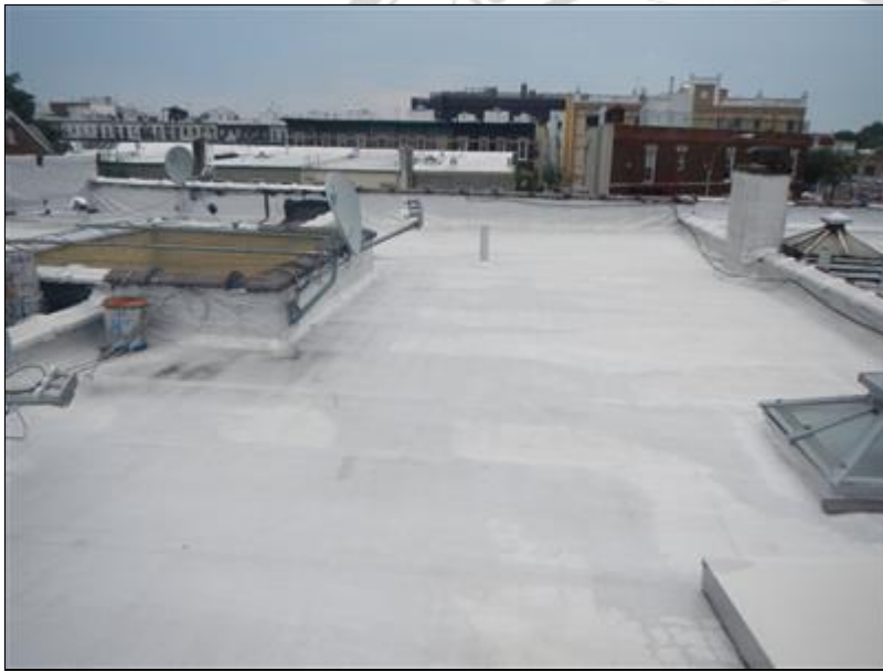
1.3 Picture 2 Roof View toward rear, no vents visible
