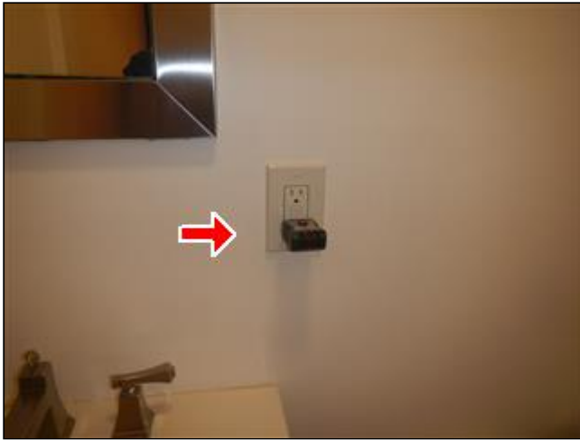
5.5.B Picture 1 Outlet has no current
