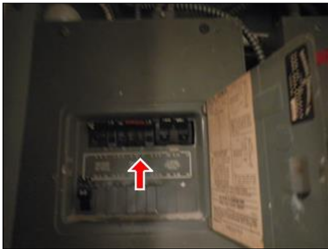
8.6 Picture 4 Second floor panel
