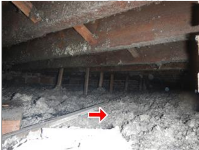
1.7 Picture 2 blown in insulation
